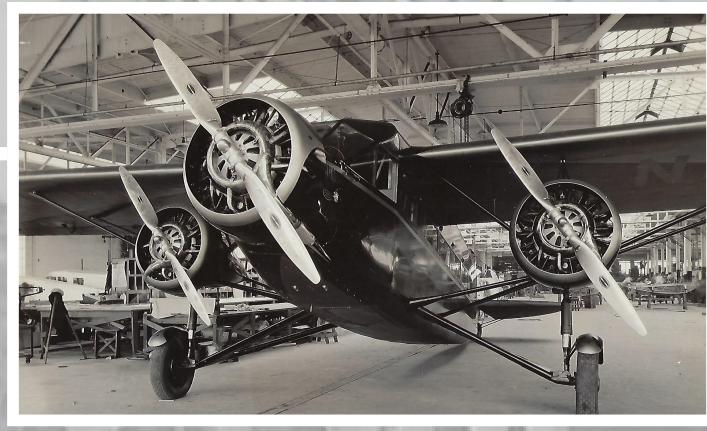
The company also made some of the first passenger planes. This SM-6000 Tri-Motor could hold II passengers and was bought by new airlines like Delta and American Airways.
